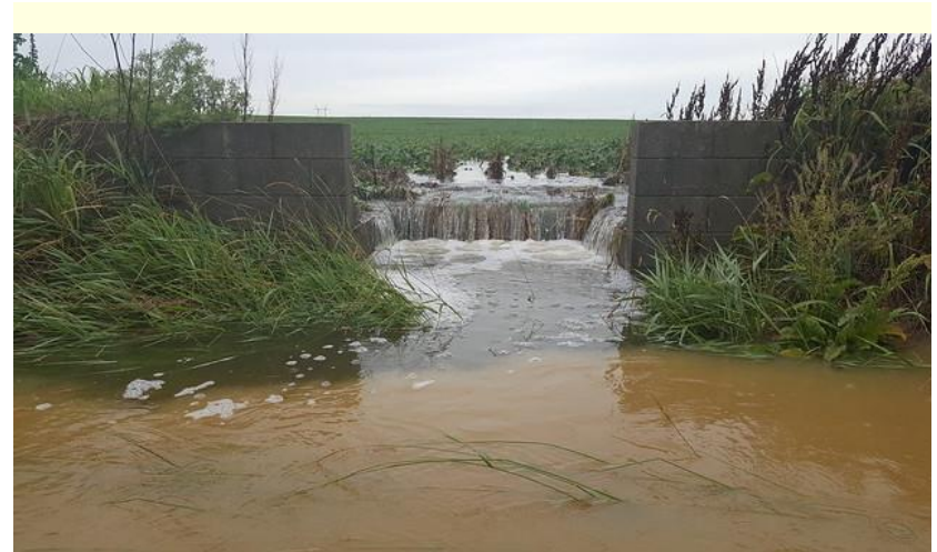
Clear runoff from cover-cropped, no-till soybean field. Note muddy water in foreground, clear water running off field. June 23, 2017, Gibson Co., IN Photo credit: SW Indiana USDA-NRCS
